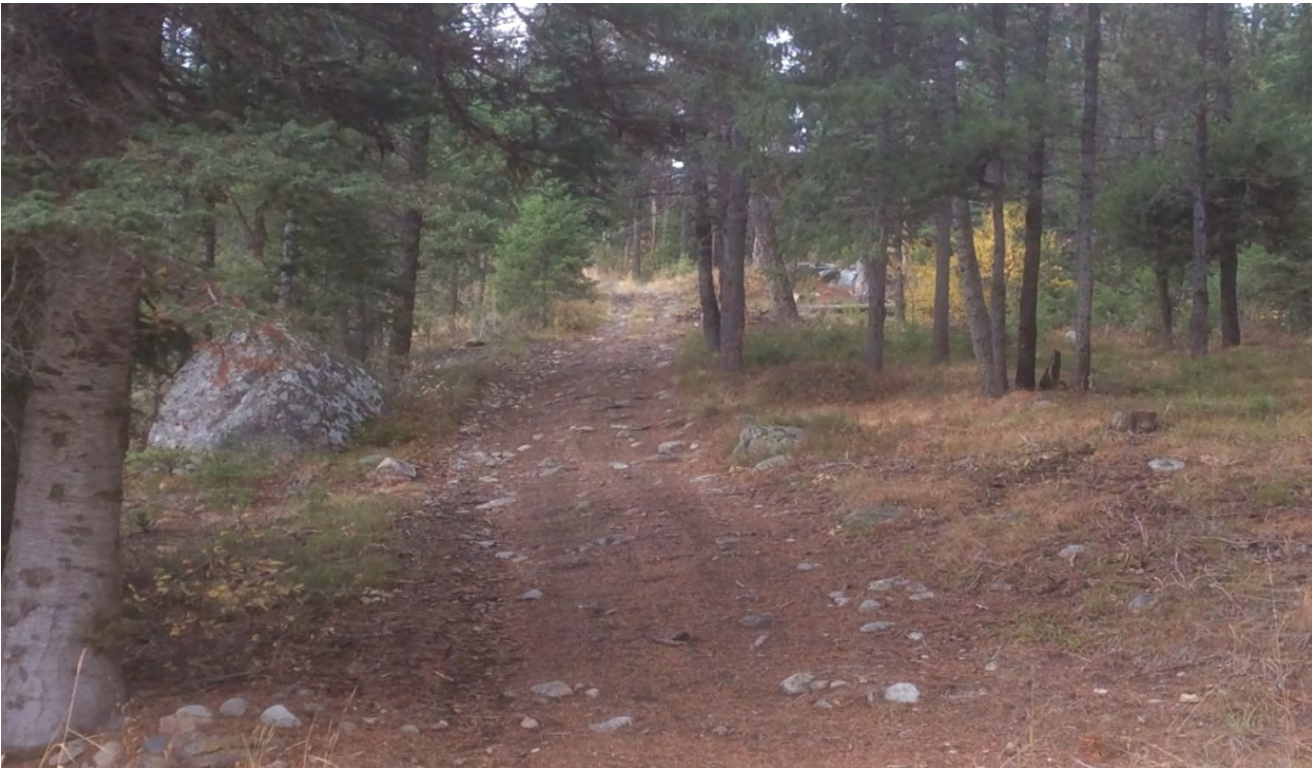
12' wide right-of-way for the buried 1340' of 4" penstock and steep ATV access trail to the diversion
